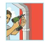
MEASURE the end of the gutter and attach a down-spout redirector or plastic flex hose that fits correctly and will reach to the barrel.
